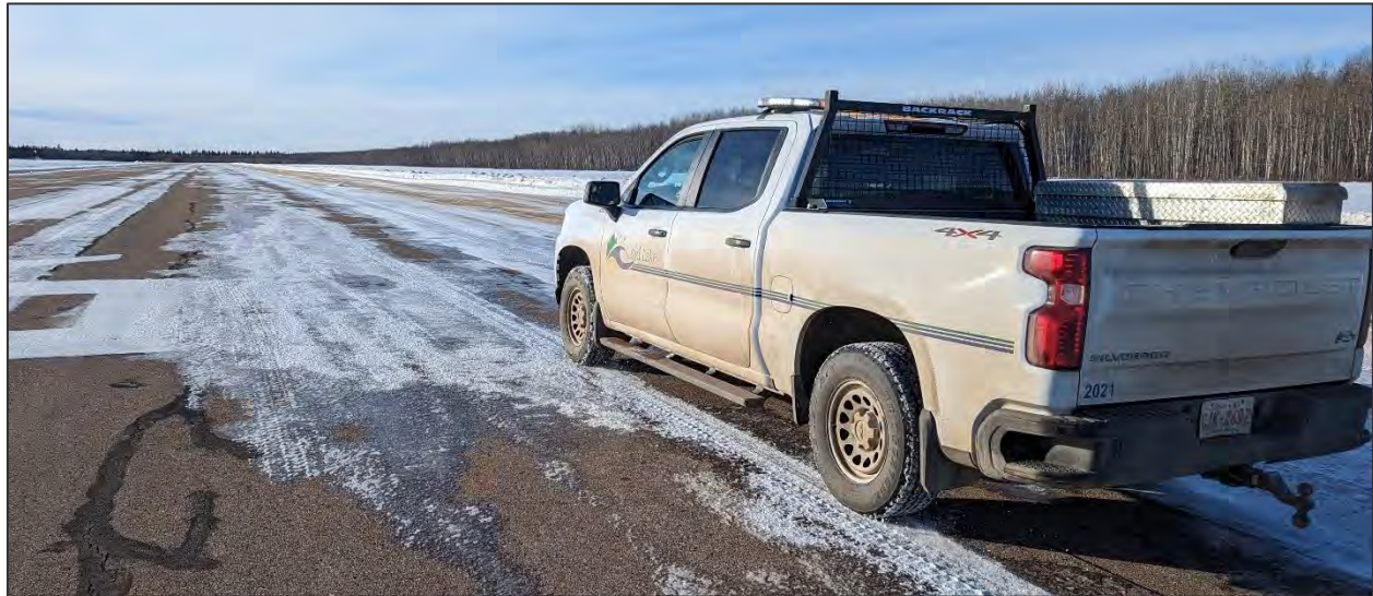
Runway inspection at Cold Lake Regional Airport
